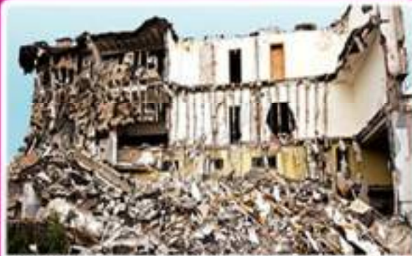
STRUCTURAL COLLAPSE (Building collapse)
